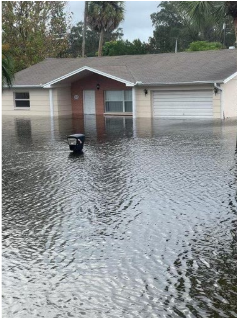
Figure 1. Storm Surge impacting a residential home along Pasco County's coastline
