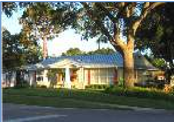
Single-family Dwelling in Downtown Neighborhood
