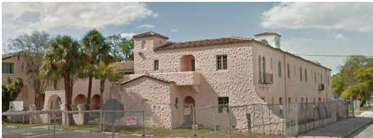
Figure 14: Hacienda Hotel (southeast corner)
