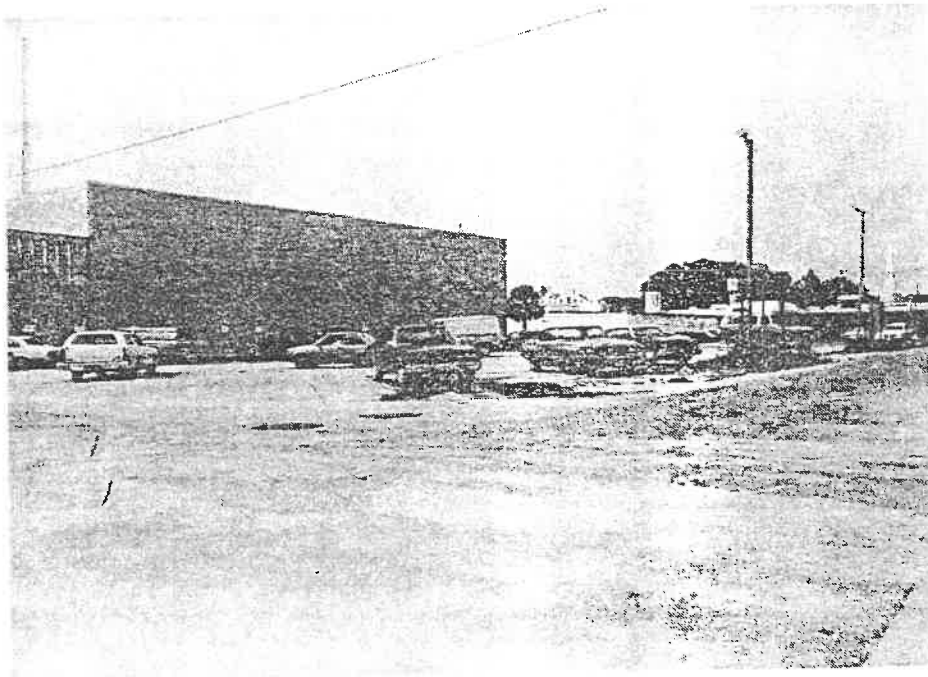
N.W. corner of Adams and Missouri, showing the lack of curbs, sidewalks, and landscaping. Without trees, the parking lot is barren.
